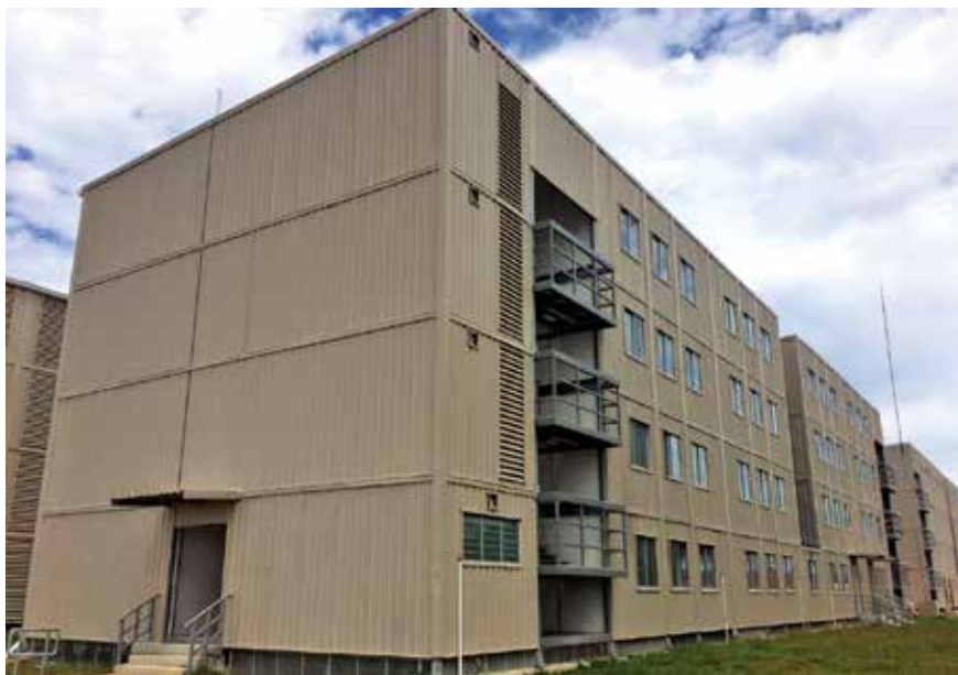
RAPID Workers' Village, Pengerang, Johor
