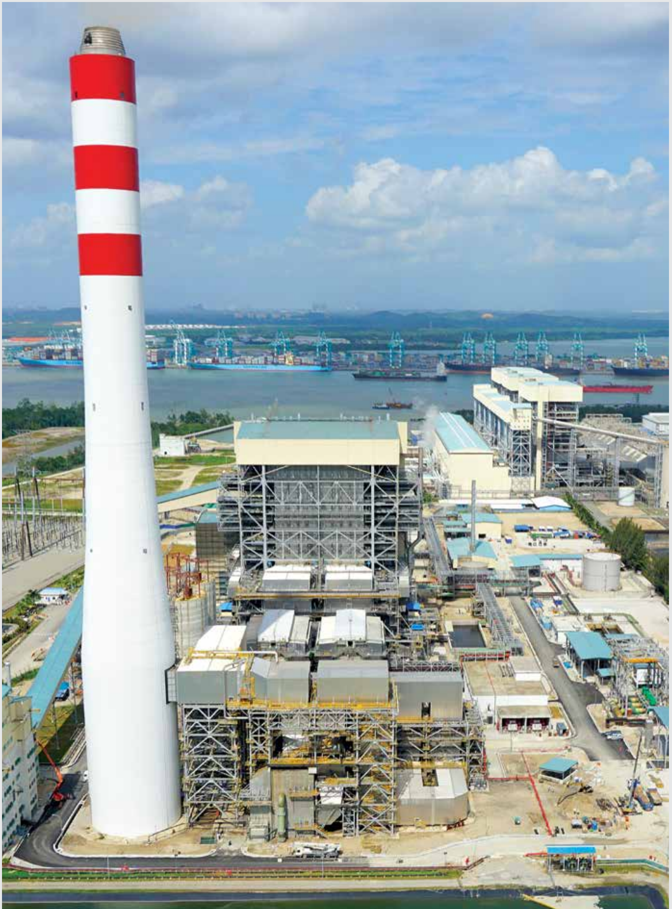
1 x 1000MW Net Coal-Fired Ultra-supercritical Power Plant, Tanjung Bin
