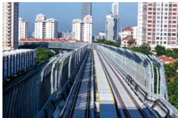
Mass Rapid Transit (MRT) V3 Viaduct Work Package from Dataran Sunway to Section 17
