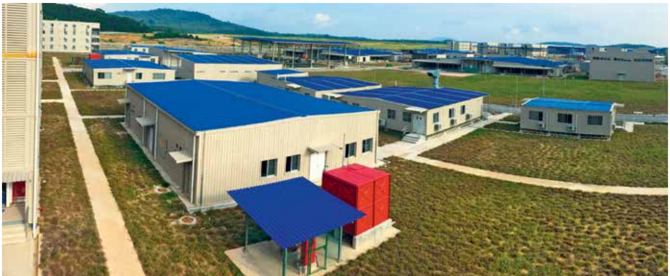
RAPID Workers' Village, Pengerang, Johor
