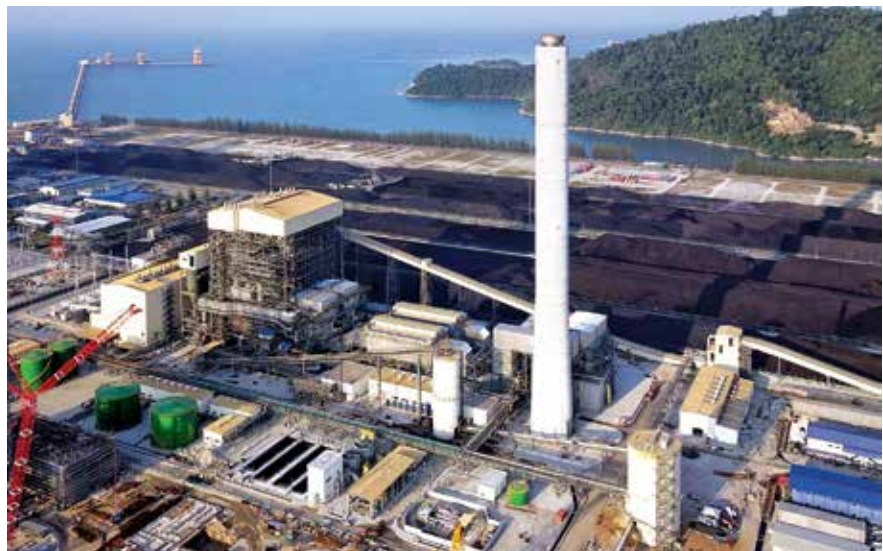
1,000MW Manjung 4, Southeast Asia’s First Ultra-supercritical Coal-fired Power Plant, Manjung, Perak
