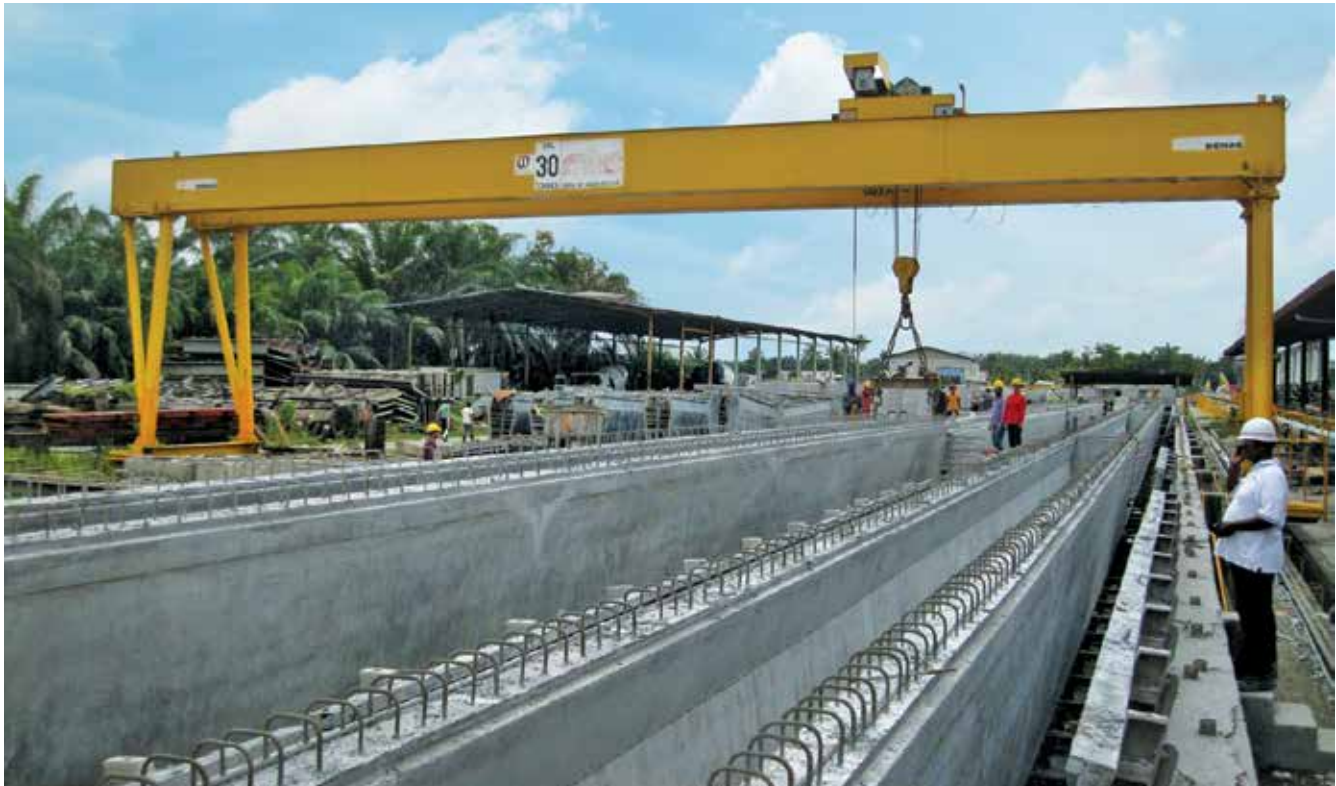
Precast Manufacturing Plant in Mukim Ijok, Selangor
