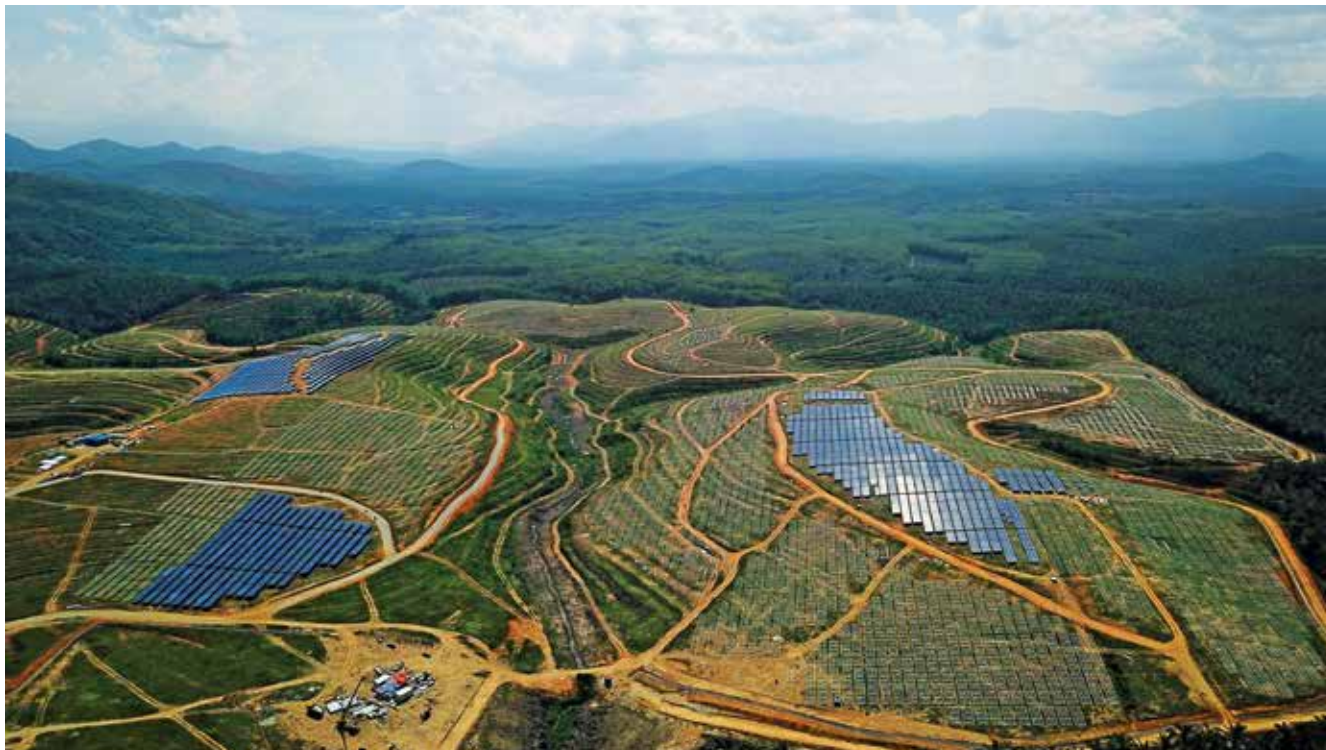
49MWa.c. Large Scale Solar Photovoltaic power plant (LSSPV), Sungai Siput, Perak
