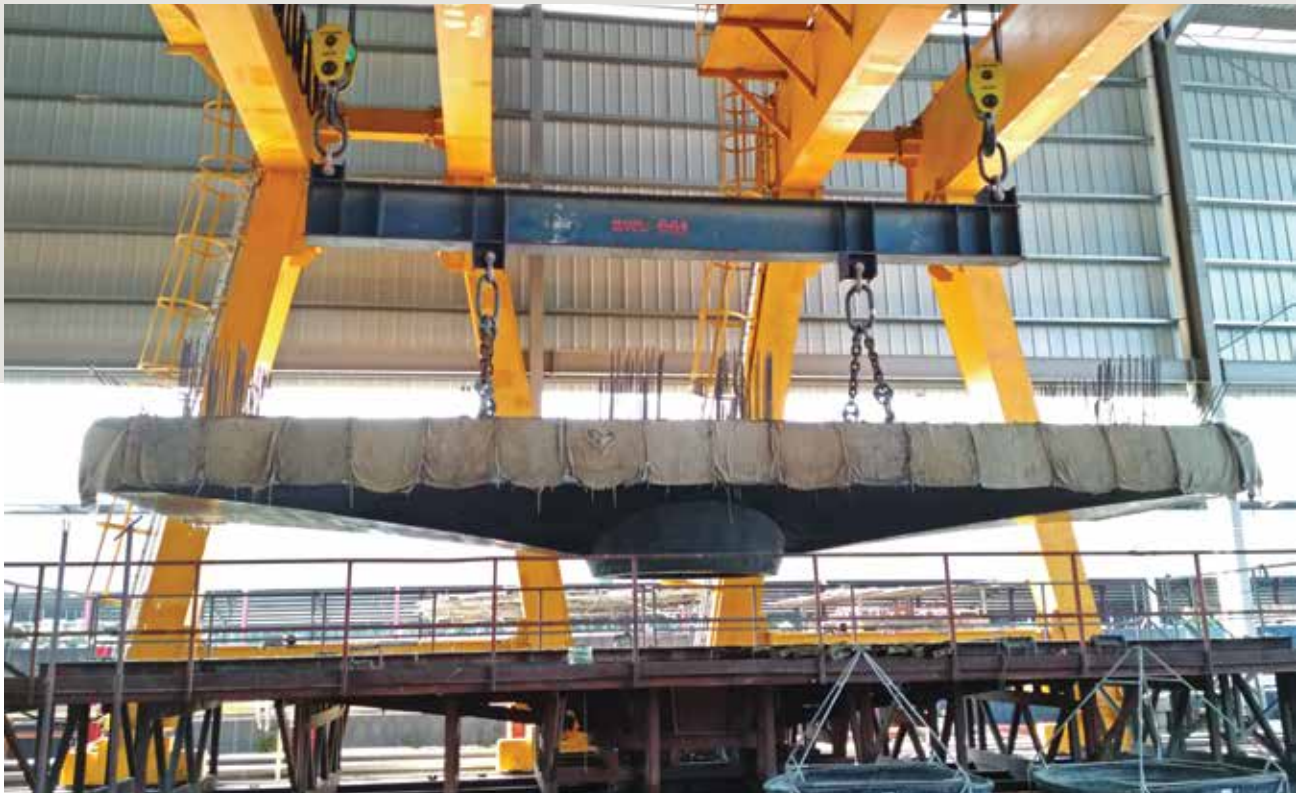
MJC Precast Sdn Bhd – Casting of Pier Cap for LRT 3 Project
